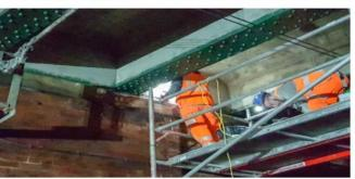
**The outcome:** The repair and strengthening works to the soffits of Golborne Railway Bridge were completed despite repeat interruptions from train movements as well as numerous
