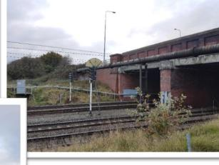
APA Concrete Repairs Ltd were successful in their tender bid and appointed as Principal Contractor to undertake concrete repairs and a carbon fibre wrap containment to the bridge soffits.
